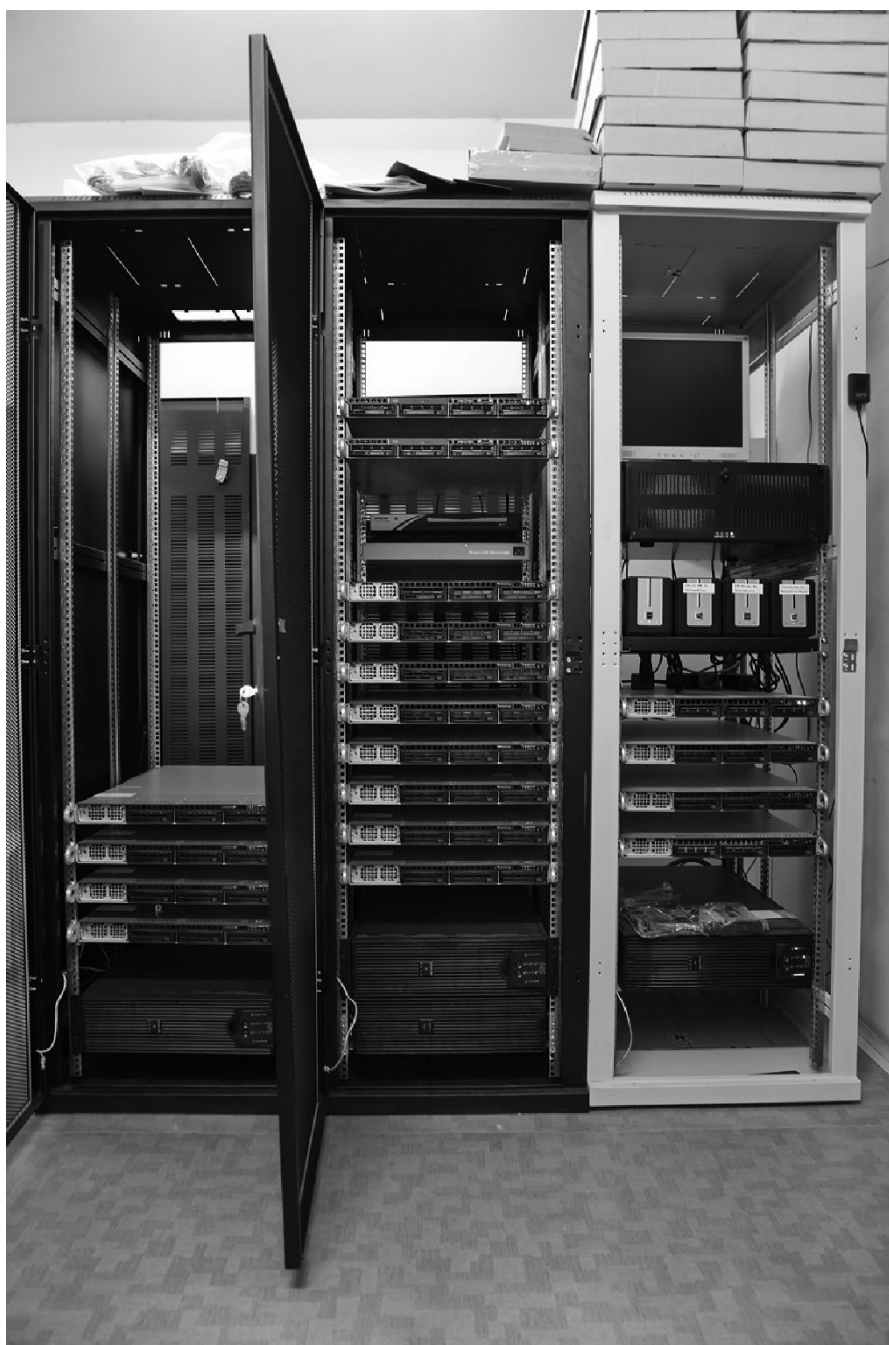
Figure 5. Constructing the cluster (november 2010).
