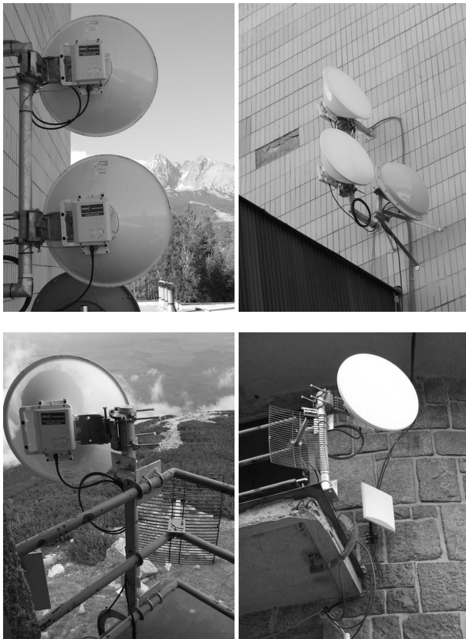
Figure 1. The antennas of the new radio interconnection at the main building in Stará Lesná and the observatory at Skalnaté Pleso.
